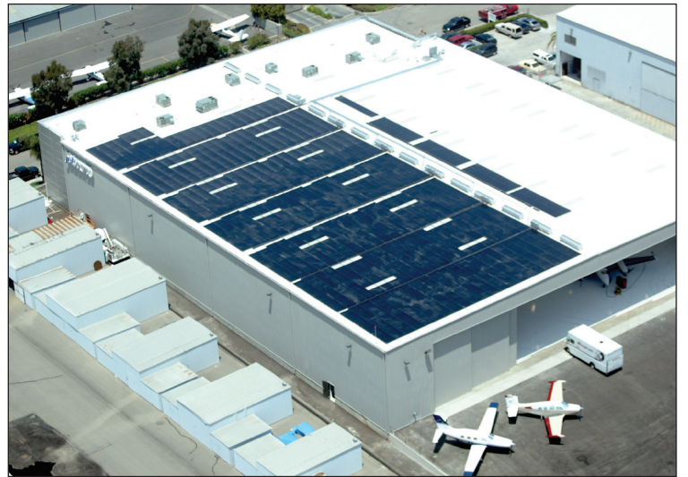
Jet Source placed SoCal's Shell Solar photovoltaic(PV) panels on its hanger roof.
